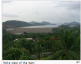
Volta view of the dam
